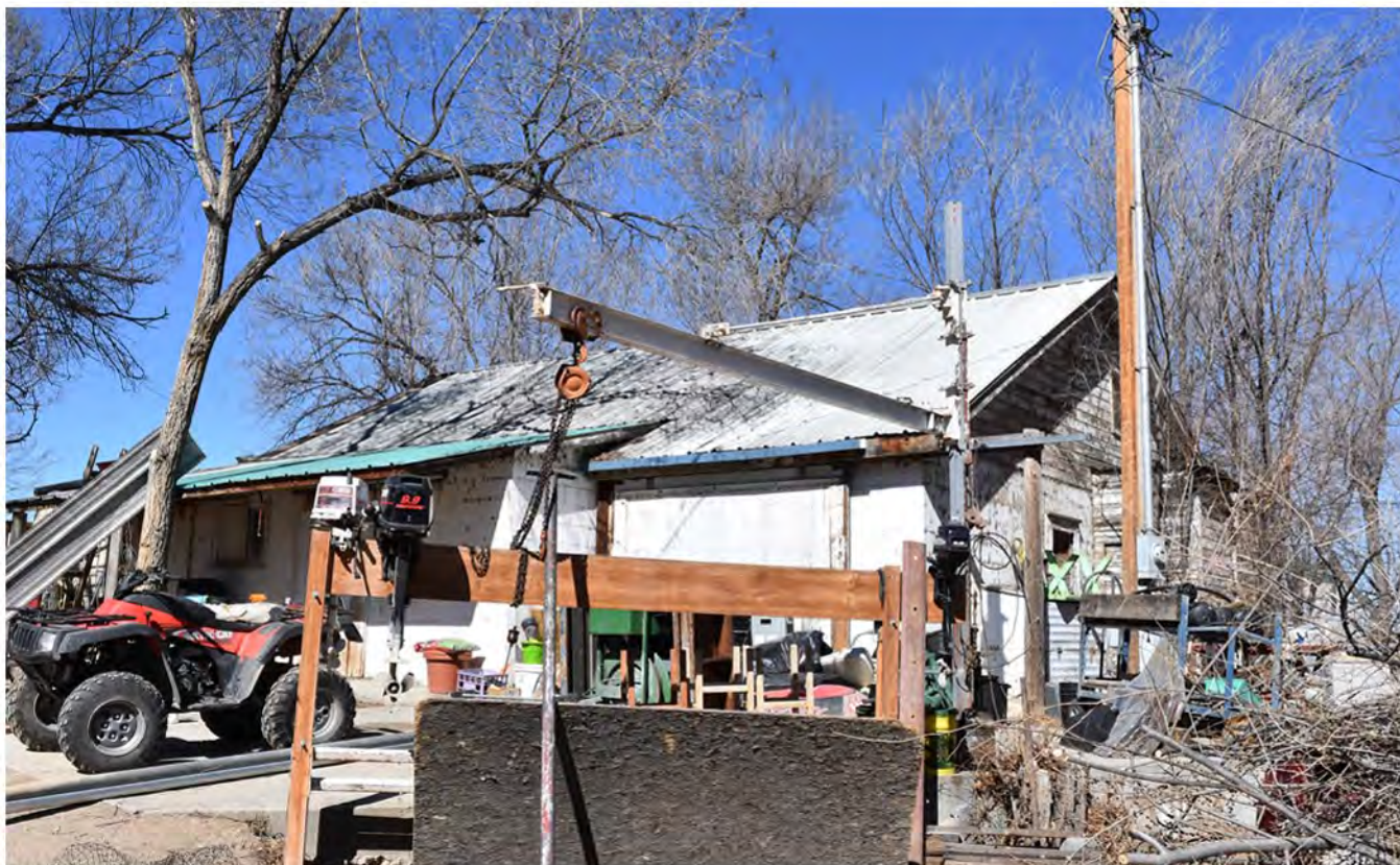
5LR14128_3: View northwest toward farm utility building built in 1930 of concrete block exterior walls.
